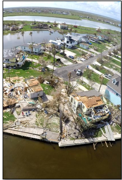
Extensive damage in Rockport, TX following Hurricane Harvey in 2017. Photo credit: AEP Texas
